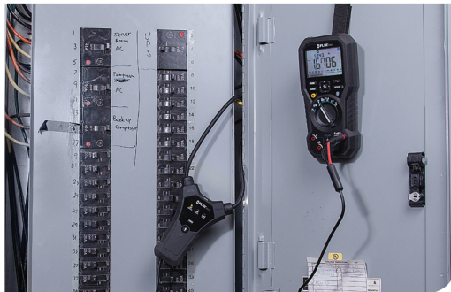
FLIR TA74 used in concert with the FLIR DM93 MultiMeter
